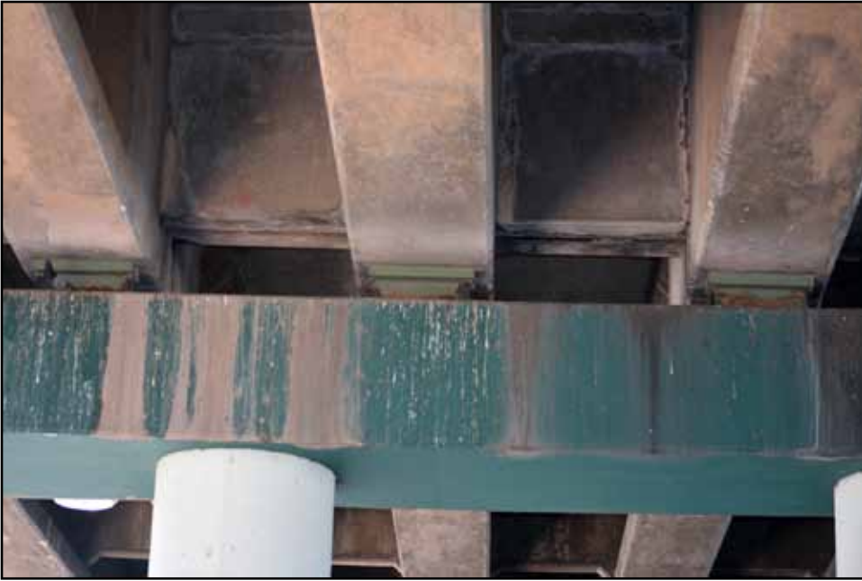
The newer traffic girders are shown supported by steel blocks.
